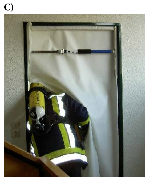
FIGURE 4: PathMaster ®; A) Door before installation of the device, B) Installation of a PathMaster ®, C) Easy access for firefighters to the fire area.
