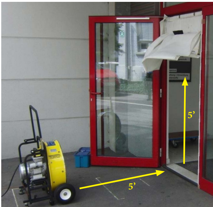
FIGURE 21: Using a PathMaster ® in the entrance door of a building increases the differential pressure and helps to show personnel present that this access is blocked by the fire department.
