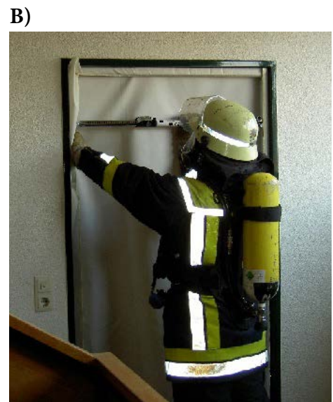
FIGURE 4: PathMaster ®; A) Door before installation of the device, B) Installation of a PathMaster ®, C) Easy access for firefighters to the fire area.
