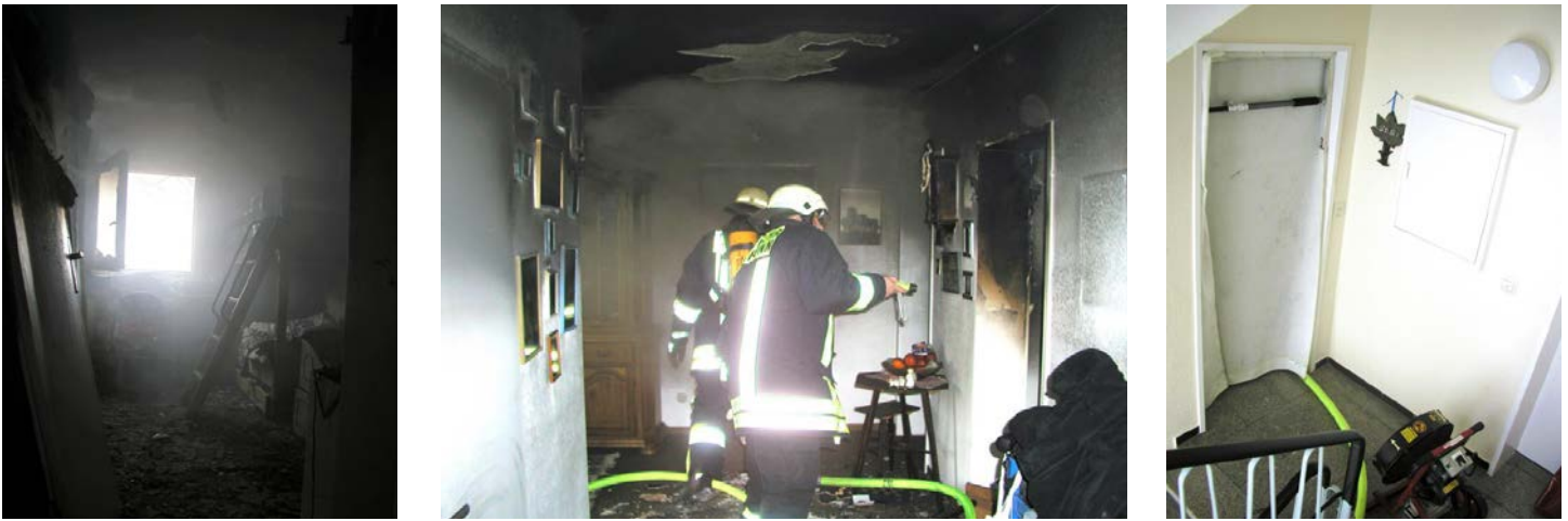
FIGURE 5: Fire in a multi-story dwelling in Heilbronn, Germany (Feb. 6, 2006). The fire room was totally damaged and the corridor was considerably damaged by heat and smoke. Meanwhile, the stairway was protected efficiently by deploying a PathMaster® .
