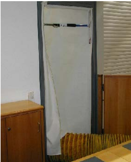
FIGURE 15: Room fire at an airport terminal in Stuttgart. To prevent smoke from spreading during the ventilation process, the door can be closed with a PathMaster®.
