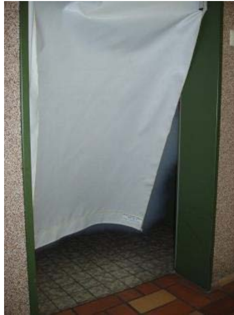
FIGURE 11: A PathMaster® makes airflow visible. The movement of air into a fire area can be seen and a safe view into the room can be facilitated by using a PathMaster®.
